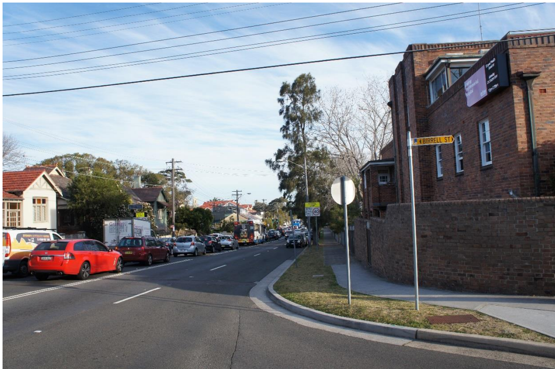
d) View looking south along Carrington Road at the corner of Birrell Street.
